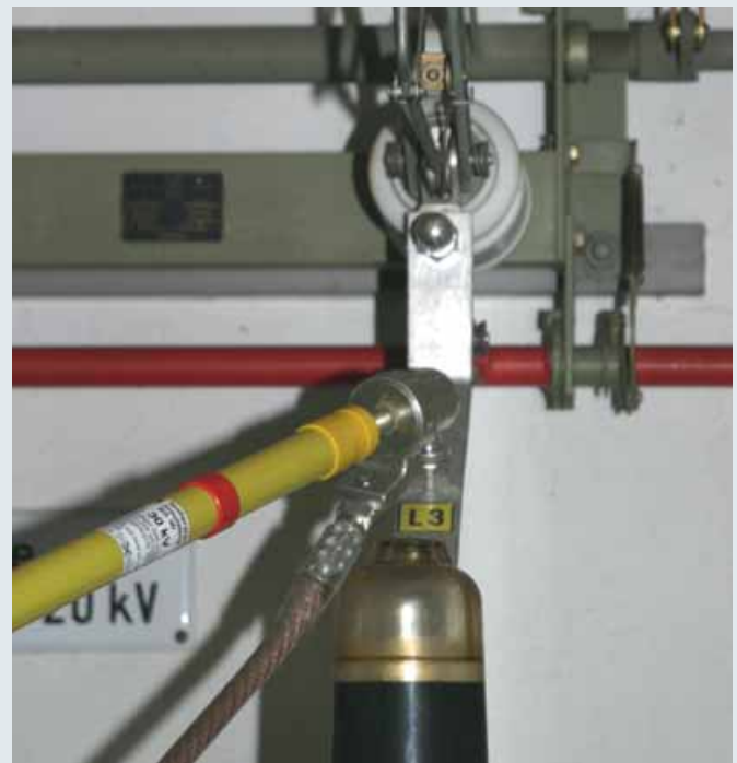
IS SK insulating stick used for clamps with hexagon shaft of earthing and short-circuiting devices.
