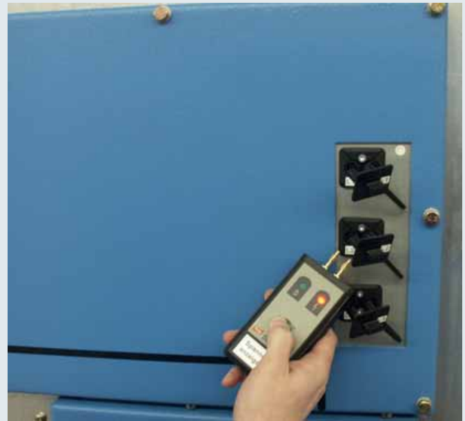
Self-test of a DEHNcap/A voltage indicator
