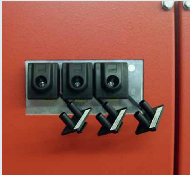
DEHNcap/P passive voltage indicator used in an encapsulated switchgear installation
