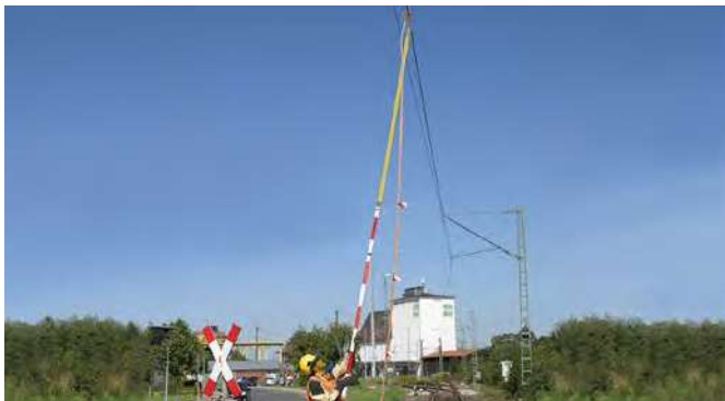
Attaching a railway earthing device.
